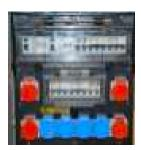
Electricity panel "type B" 2 × CEE / 32 (400 V) 2 × CEE / 32 (400 V) 4 × T25 / 16 (400 V) Total 63 A
