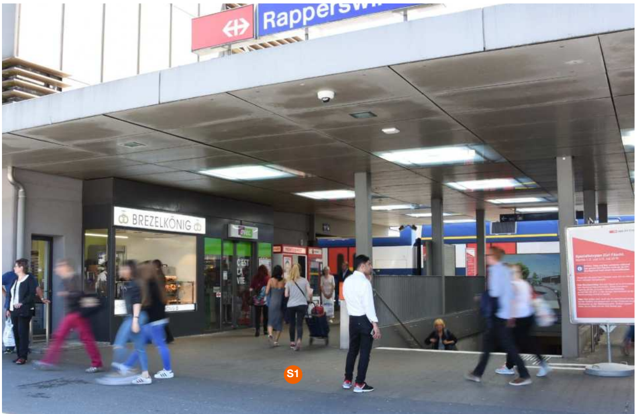
At pedestrian underpass, city level
