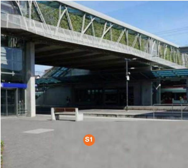
S1 Station square, Passage West
