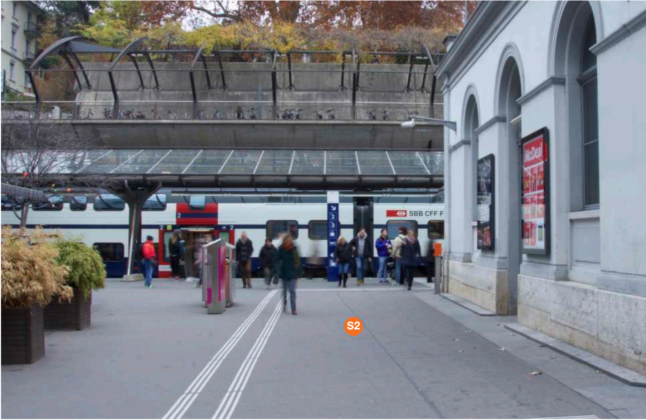
S2 Distribution point, Passage west
