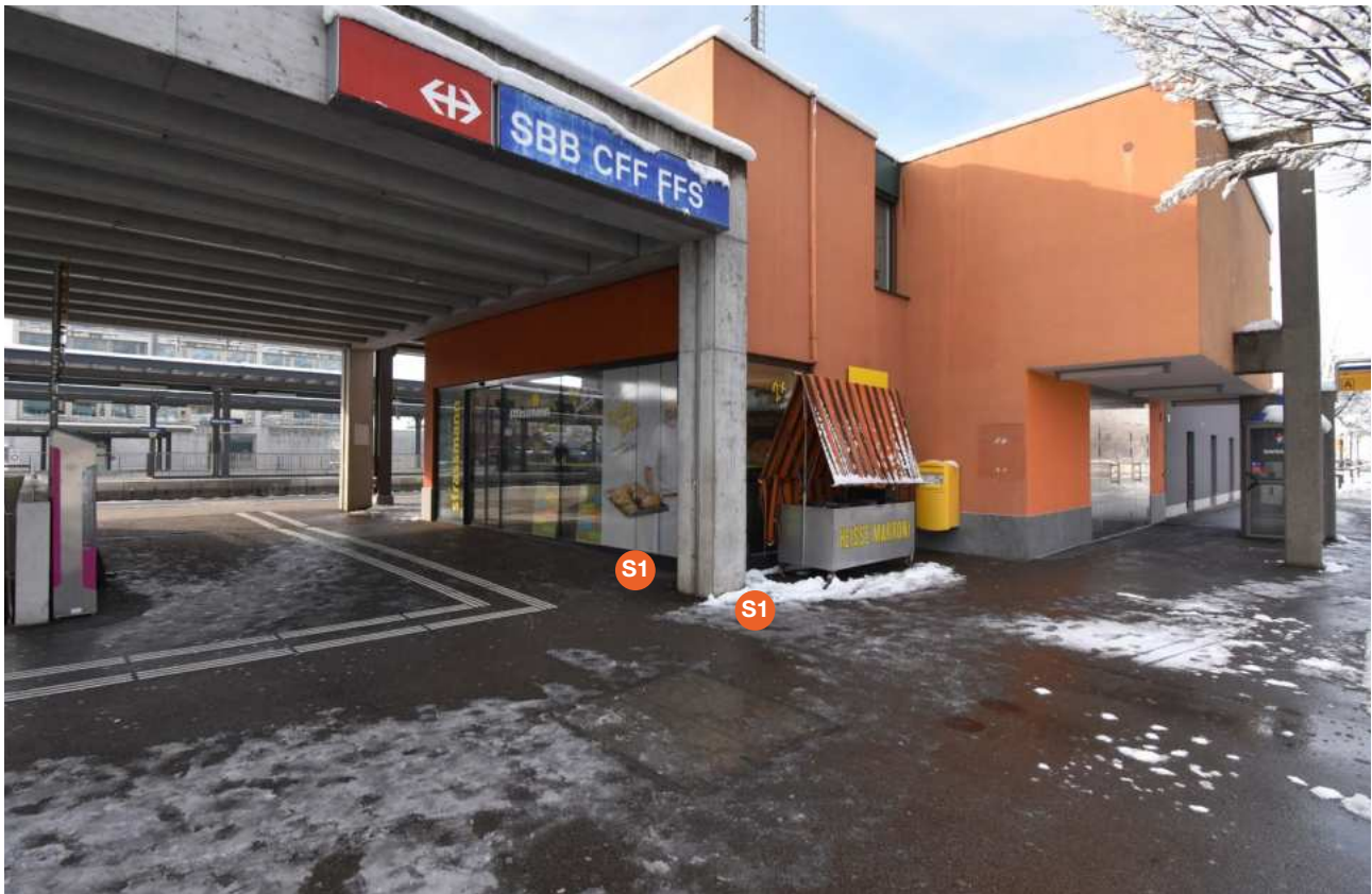
Covered sampling point, in rain and snow / Uncovered sampling point, in dry weather conditions
