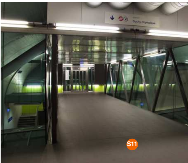
Station Fourmi, on both sides of the track crossing. Access to both platforms
