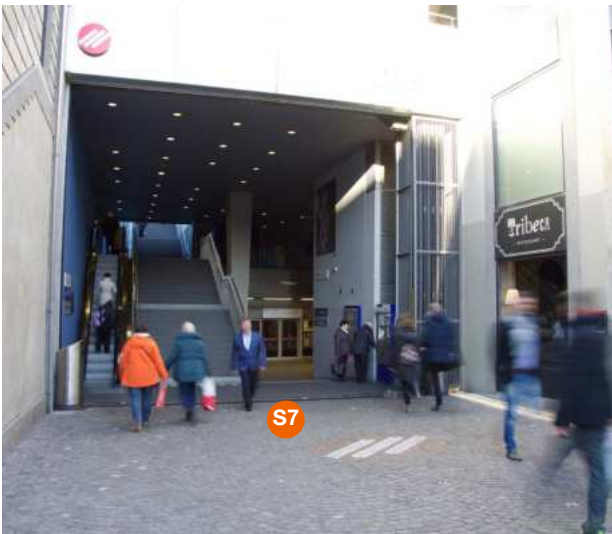
Station Riponne-M. Béjart, on the side of Place Arlaud.
