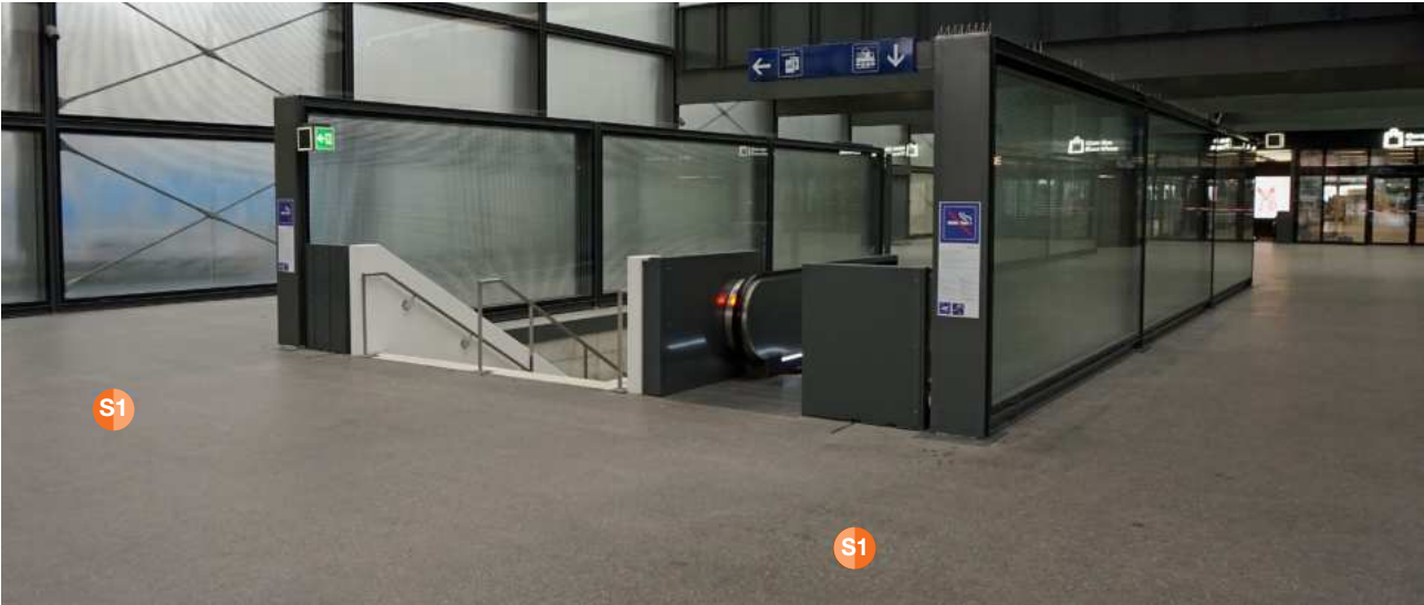
S1 2 half distribution points, Genève Eaux-Vives - West entrance, city level, in front of the escalator
