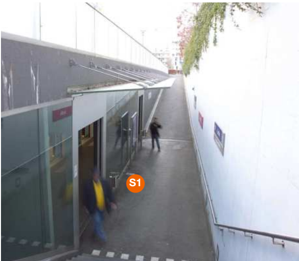
Station Jordils, entrée est, direction Croisettes
